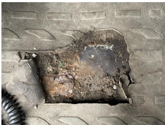
2: Carpets Front Torn Over 10mm
